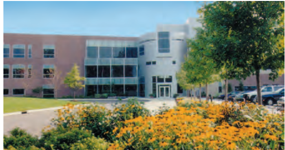
Parker Hannifin Corporation Headquarters Cleveland, Ohio
